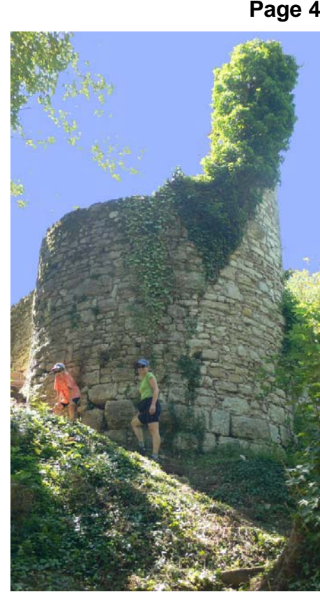
Dominick thought this castle ruin in Ferrette was too "ruined"
